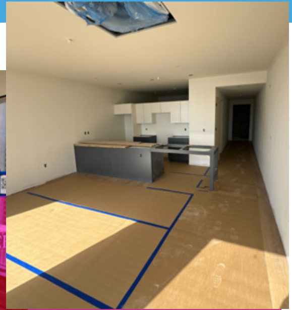
150 E. Gay conversions under construction, The Bernstein Companies
