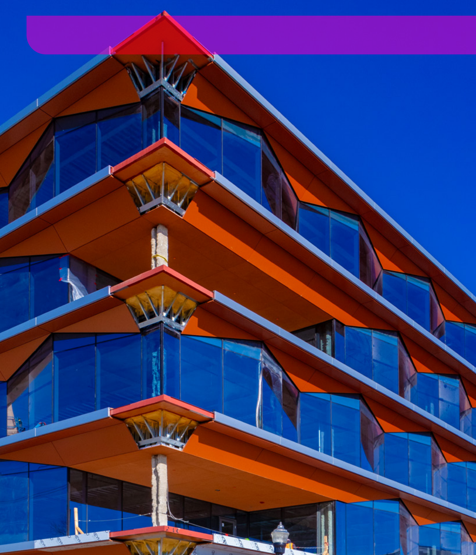
Astor Park Office under construction, Andy Spessard
